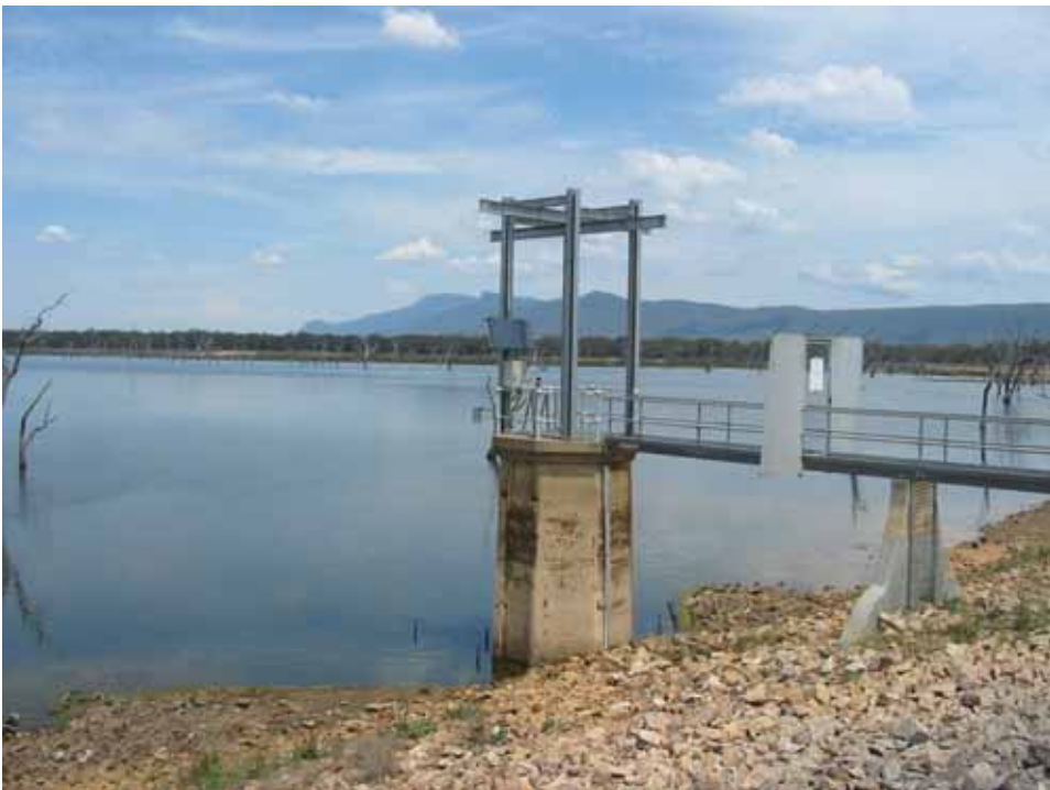
Lake Fyans Water Supply Outlet Tower (photo – G. Saunders)
